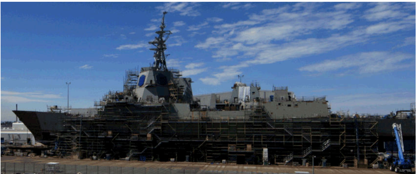
Figure S.1: The future HMAS Hobart under construction, December 2013
